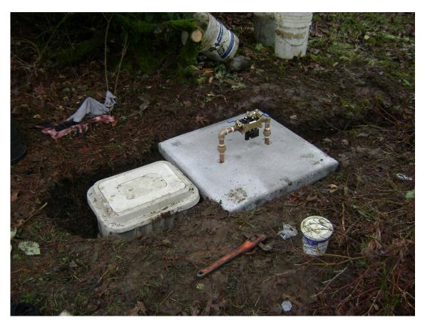
The below image shows the completed setup with the water meter, the device, the device pad and the backflow box installed.
