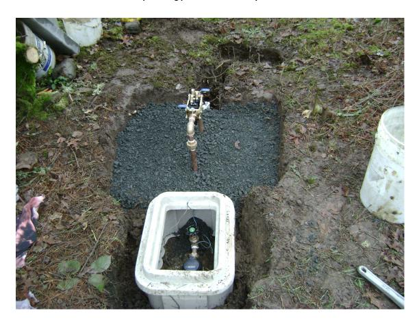
The below image shows the water meter, the device and the device pad installed. Notice the clearance between the drain ports on the backflow device and the backflow pad.
