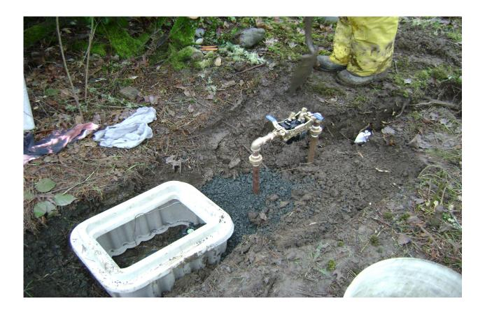
The below image shows the water meter and the device installed with crushed rock around the base of the plumbing parts to add stability for the device.
